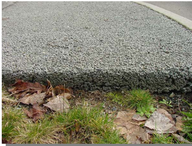
Figure 630.9 Porous concrete sidewalk cross-section, in Olympia
