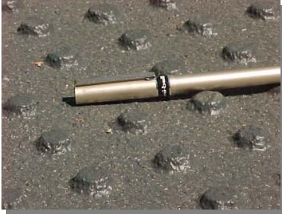
Figure 630.4 Close-up of truncated domes with pen for scale
