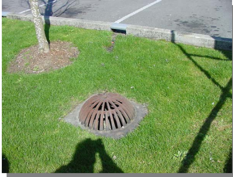
Figure 630.7 Inlet for subsurface drainage
