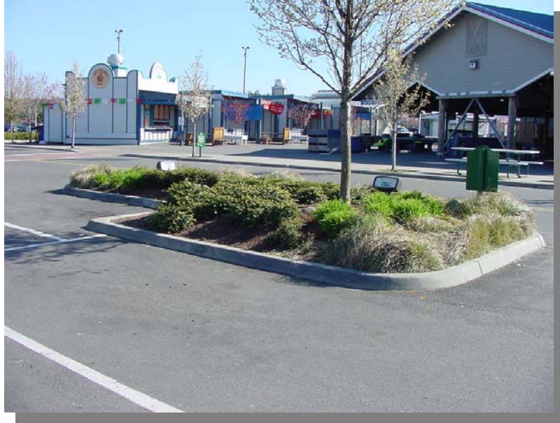
Figure 630.11 Raised curbs around end island
