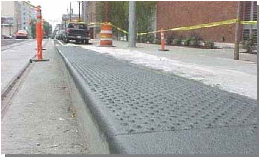
Figure 630.3 Truncated Domes under construction at transit stop
