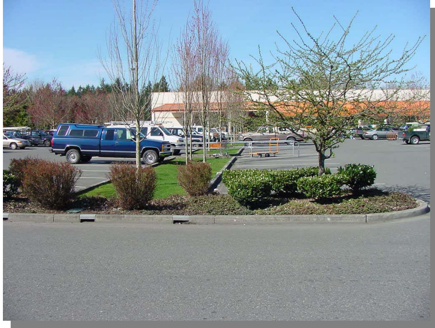
Figure 630.5 Vegetated bioswale in parking lot
