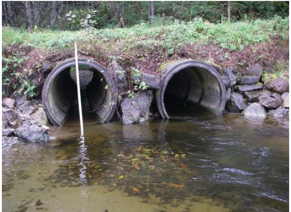
Above: Jansen Creek culvert at SR 112 before it was corrected by WSDOT in 2016. This project is applicable to the 2013 federal injunction. Below: The same location after WSDOT corrected the culvert using bridge design methodology. This design allows unhindered passage for fish to reach quality spawning and rearing habitat, and improves estuary function.
