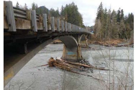
The US 101 bridge over the Elwha River.
