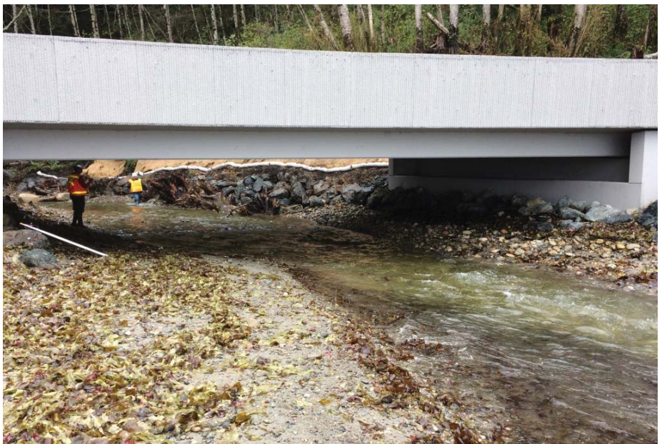
Above: Jansen Creek culvert at SR 112 before it was corrected by WSDOT in 2016. This project is applicable to the 2013 federal injunction. Below: The same location after WSDOT corrected the culvert using bridge design methodology. This design allows unhindered passage for fish to reach quality spawning and rearing habitat, and improves estuary function.
