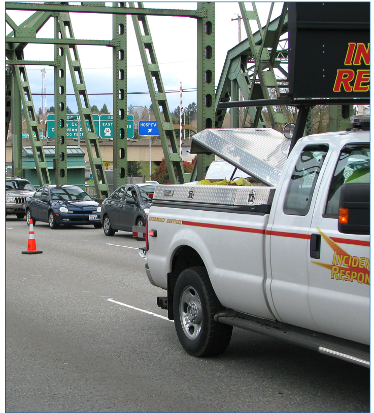
Traffic backs up on the I-5 bridge following a collision.
