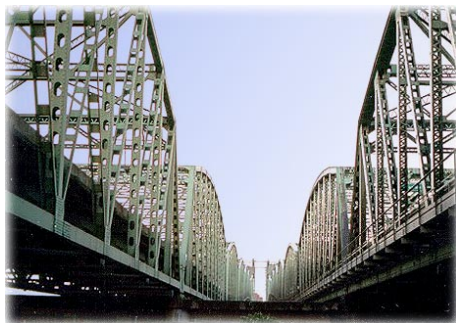
The Interstate Bridges
